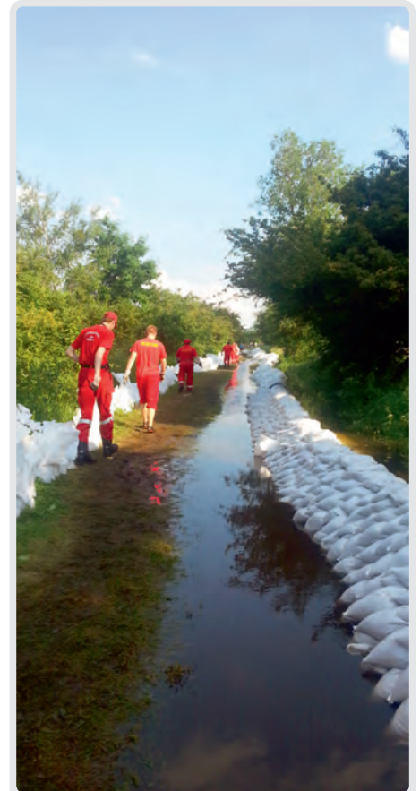
Deichsicherung in Lostau
